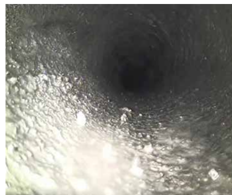
Trial hole using AMC BORE HOLE STABILISER
