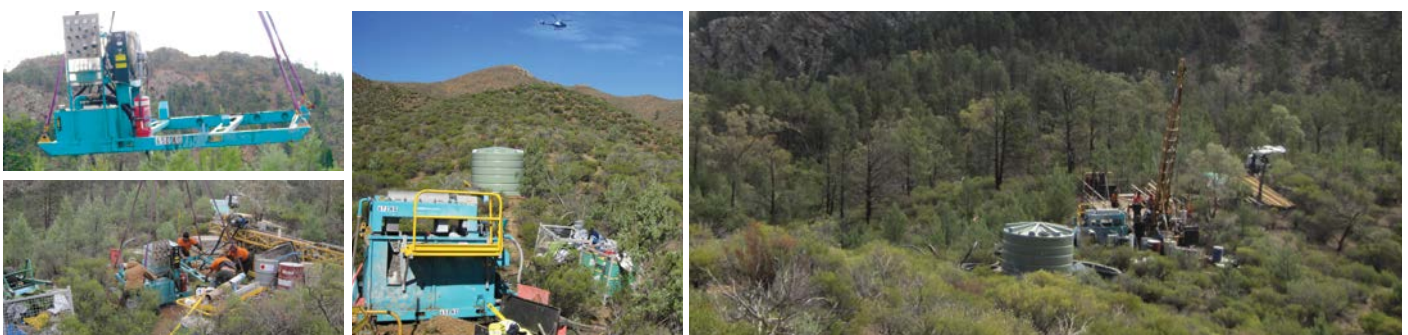
Lift and swing HP-SRU into place in difficult sloped terrain
