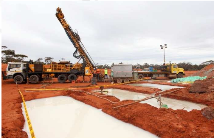
Traditional drilling fluid sumps
