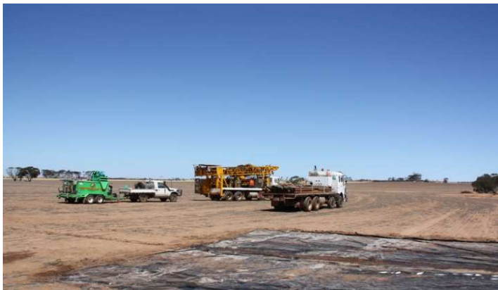
No environmental damage
