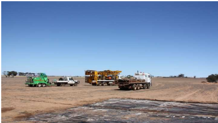
No environmental damage
